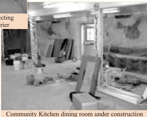
Community Kitchen dining room under construction
