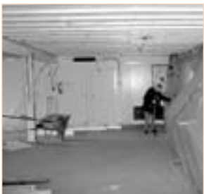
Judy Woods inspecting kitchen dust barrier
